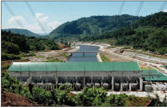
The Nam Theun 2 powerplant in Lao PDR, the country's largest scheme. It supplies electricity to EGAT in Thailand.
