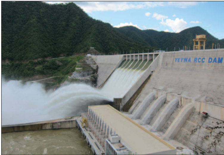
Myanmar's 790 MW Yeywa hydro station on the Myitnge river, the country's largest hydro plant in operation to date.
